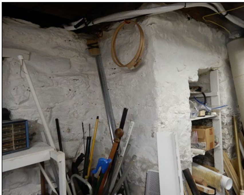
Photo 21. Frame-plank house end wall basement fireplace support, view southwest.
