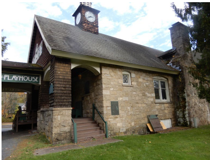
Figure 25: Shawnee Playhouse, view northeast
