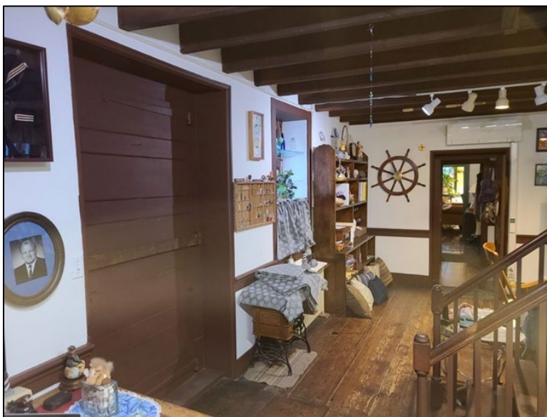
Photo 24. Stone storehouse front wall main first floor room with wide entry door, view south.
