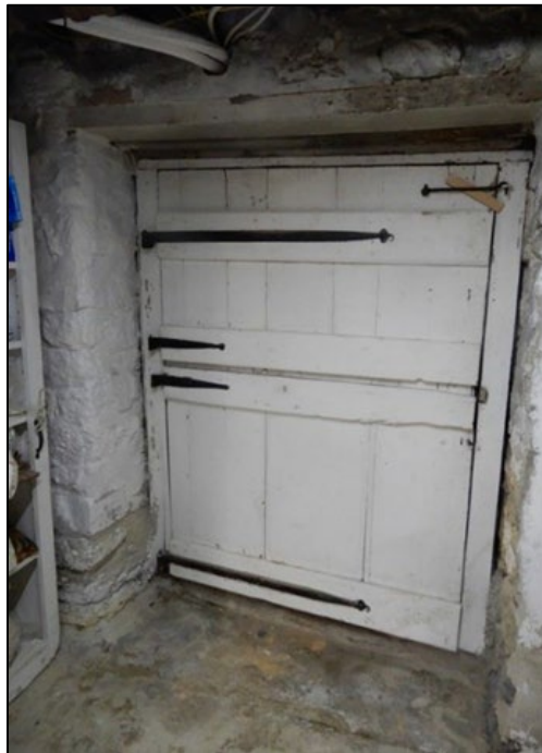
Photo 22. Frame-plank house end wall basement original exterior door, view west.
