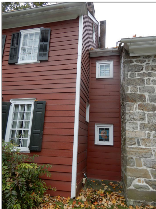
Photo 8. Frame connector built in 1943 between the frame-plank house at left and storehouse at right, view west.
