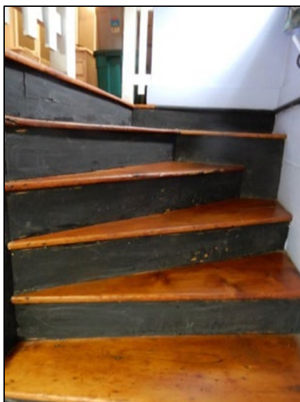
Photo 19. Frame plank house north side staircase to attic, view west.
