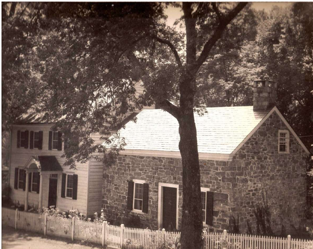
1948 House After major work
